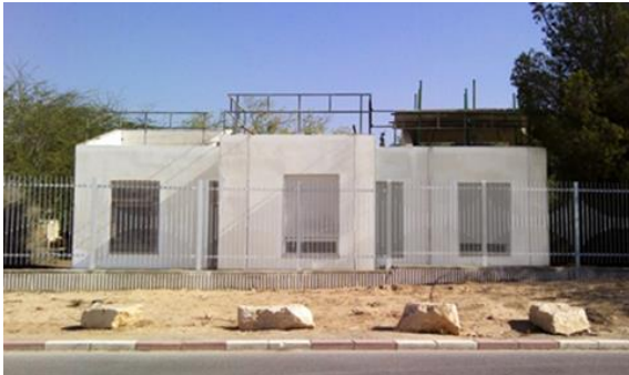
Figure 1: South façade of test building.
